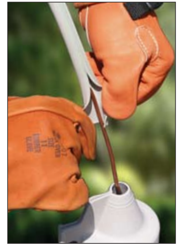
Field Installation of RUP Stinger Cover
