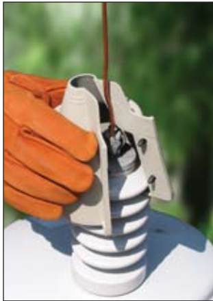
Rubber Glove Installation of R-21116
